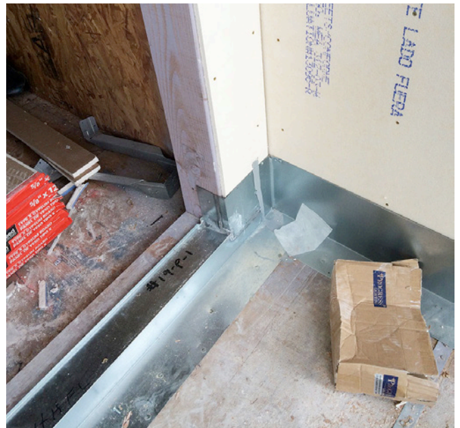
Photograph 3: Pan Flashing of Balcony Door —Note the back dam and end dam of the flashing for the balcony door. The back dam support for the pan flashing has not yet been installed. The back dam support protects the upstand of the back dam during the construction process.
