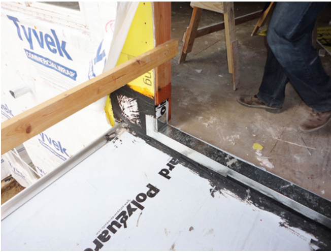
Photograph 4: Membrane Waterproofing —Additional metal flashing is installed over the waterproofing that is stripped into the pan flashed balcony door opening. This additional metal flashing protects the membrane waterproofing at the door opening.
