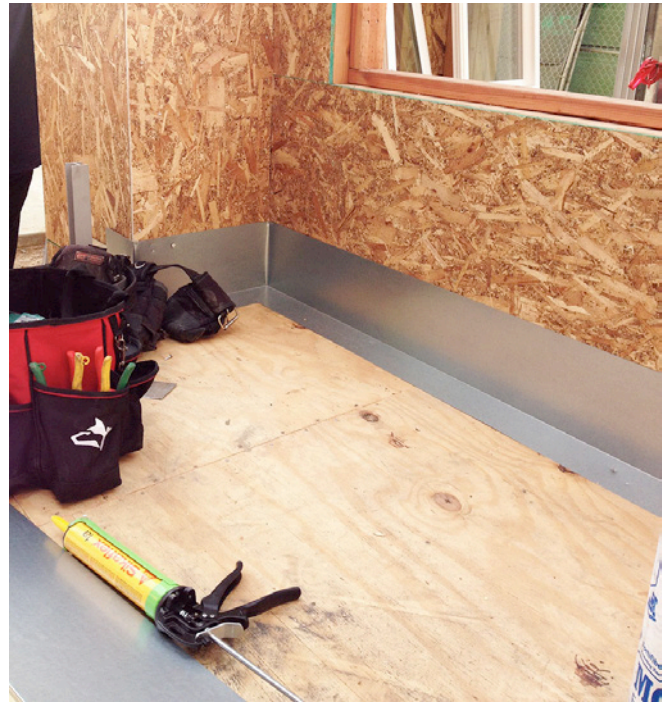
Photograph 2: Metal Angle —Note the use of plywood as the balcony deck surface. Plywood and engineered wood deck sheathing are typically both used interchangeably. However, adhesion of membrane waterproofing to engineered wood deck sheathing tends to be more difficult and primers become key to successful adhesion.
