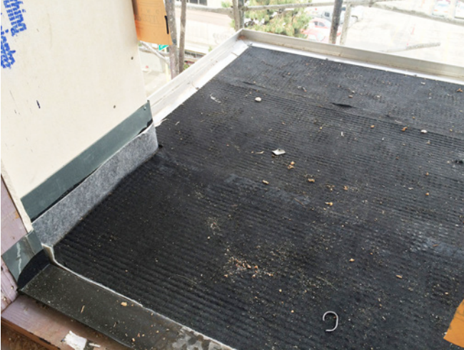
Photograph 8: More Drainage Matt —The vertical top edge of the perimeter balcony deck waterproofing membrane is yet to be stripped into the exterior wall sheathing with mastic.
