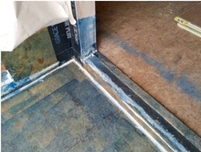
Photograph 1: Sealant Joint —A sealant joint is installed at the perimeter of the balcony deck where it intersects the exterior wall. Note the primer application on engineered wood deck sheathing and the OSB wall sheathing. The primer's function is to facilitate adhesion of the waterproofing membrane. Also note the back dam support for the yet to be installed pan flashing in the rough opening for the balcony door.
